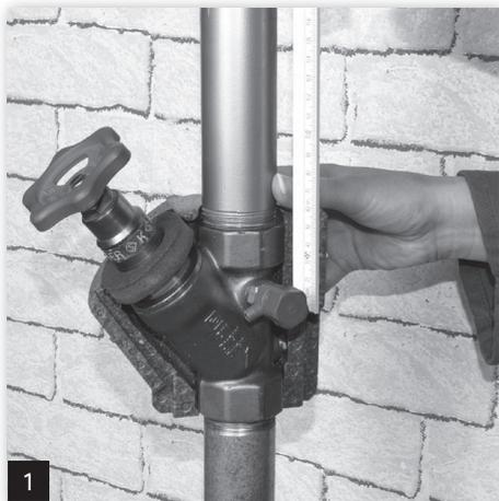
Take the measurement from the center of the discharge to the top edge of the EPP shell.
