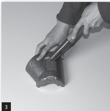
Punch out the discharge opening with a punch tool (alternatively with a cutter knife).
