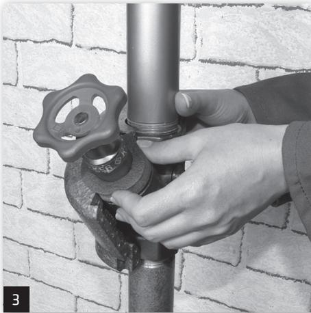
Place the first half shell and hold the adapter in position.
