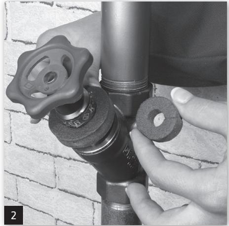
Select the appropriate soft foam adapter for the valve stem diameter.
