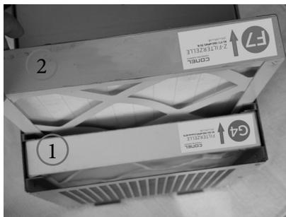
The coarse air filter, type G4, should always be used in position (1), the fine air filter, type F7, should always be used in position (2).
